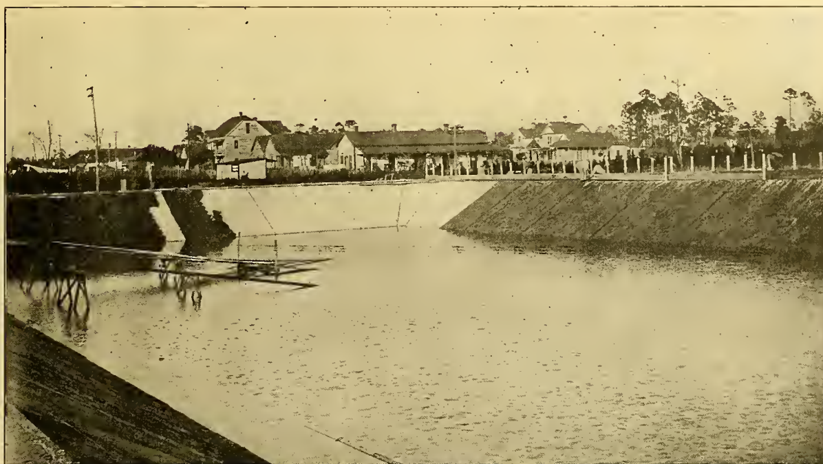
THE CITY'S NEW RESERVOIR IN COURSE OF CONSTRUCTION. When completed will hold one million gallons of water.
